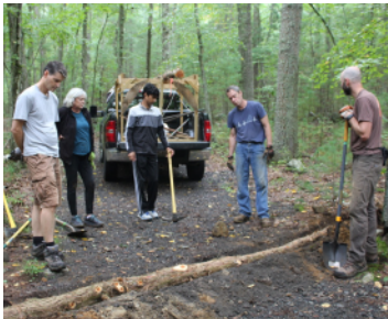
Laying new water bars
